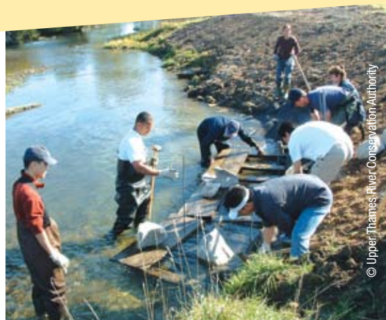
Volunteers install fish habitat on Gunn Farm
